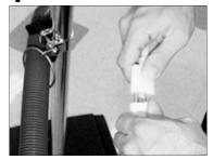
Connect the female power cord receptacle with the male plugged pigtail attached at the switch housing.
